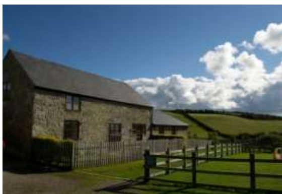
Picture 10 Converted grain storage barn
