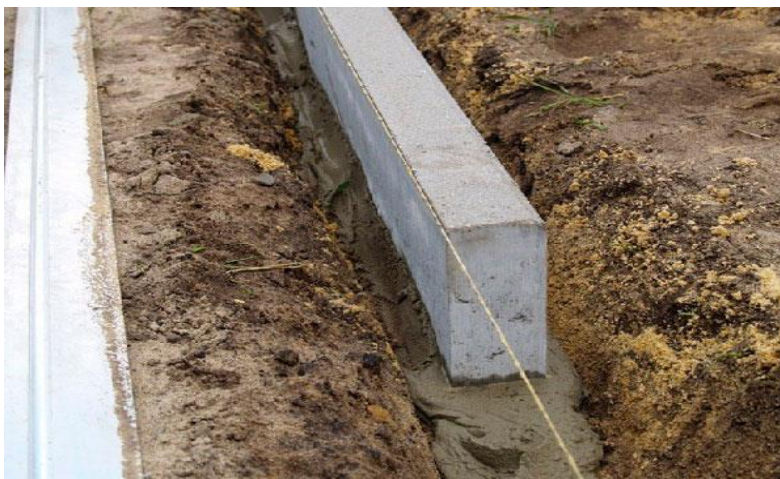
Slika 9. Primjer montaže rubnjaka (Izvor: https://tekras.ru/hr/the-construction-of-the-house/how-to-make-curbs-in-the-country-selfmade-curbs-for-the-garden-and-cottages/ )
